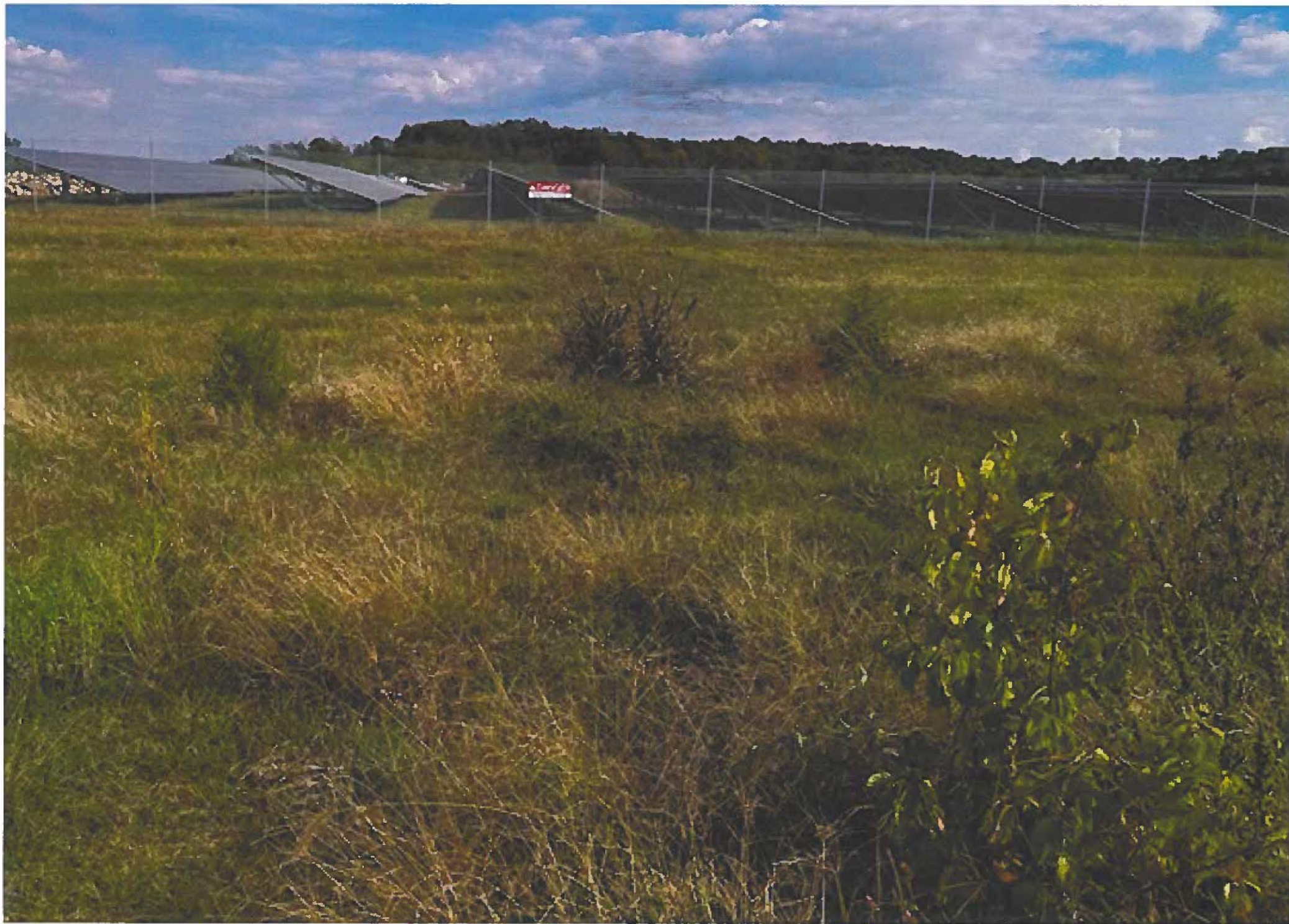
Weeds taller than trees. Road frontage. Outside of fence
